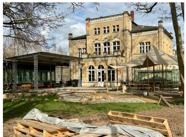
Project site in Leisnig
